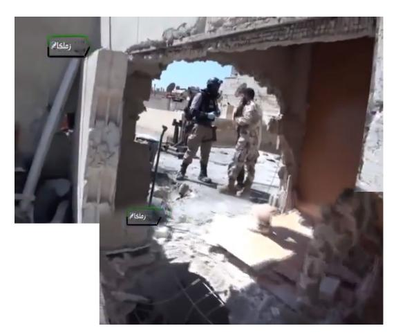
As seen in this video, and reported by the UN, the rocket penetrated the western outer wall (far wall in the photo below) and continued into the floor below. The impact force and debris likely caused the southern wall (the near wall below) to break apart.
