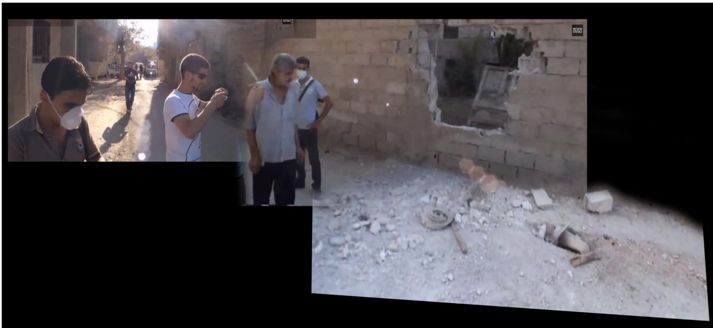
We estimate this azimuth using brick lengths. The distance from the crater to the wall is 1.8 bricks, and the rocket has landed three brick lengths laterally offset to the right of the center of the hole.
